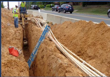
Cable Ducting Excavation
