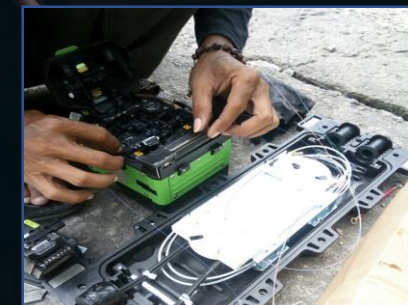
Splicing Cable on Cloure
