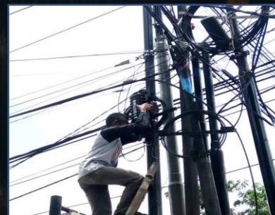
Joint Closure Installation
