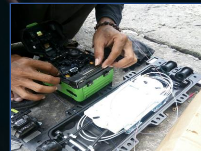
Splicing Cable on Cloure
