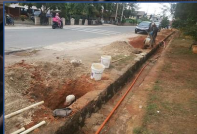
Cable Ducting Construction
